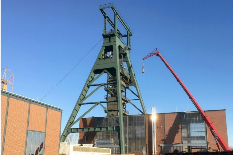
Construction site of Konrad 2 (shaft conveyor system)
