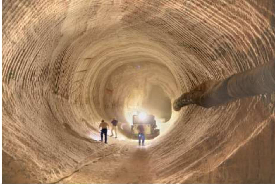
Fig. 11. Visual inspection of the location of a horizontal flow barrier in rock salt. On the right-hand side of the drift an air duct is installed to ensure ventilation.
