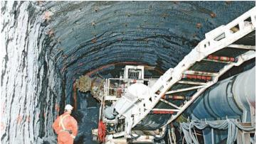
Transport drifts: anchor-shotcrete construction with steel arch support and concrete filling
