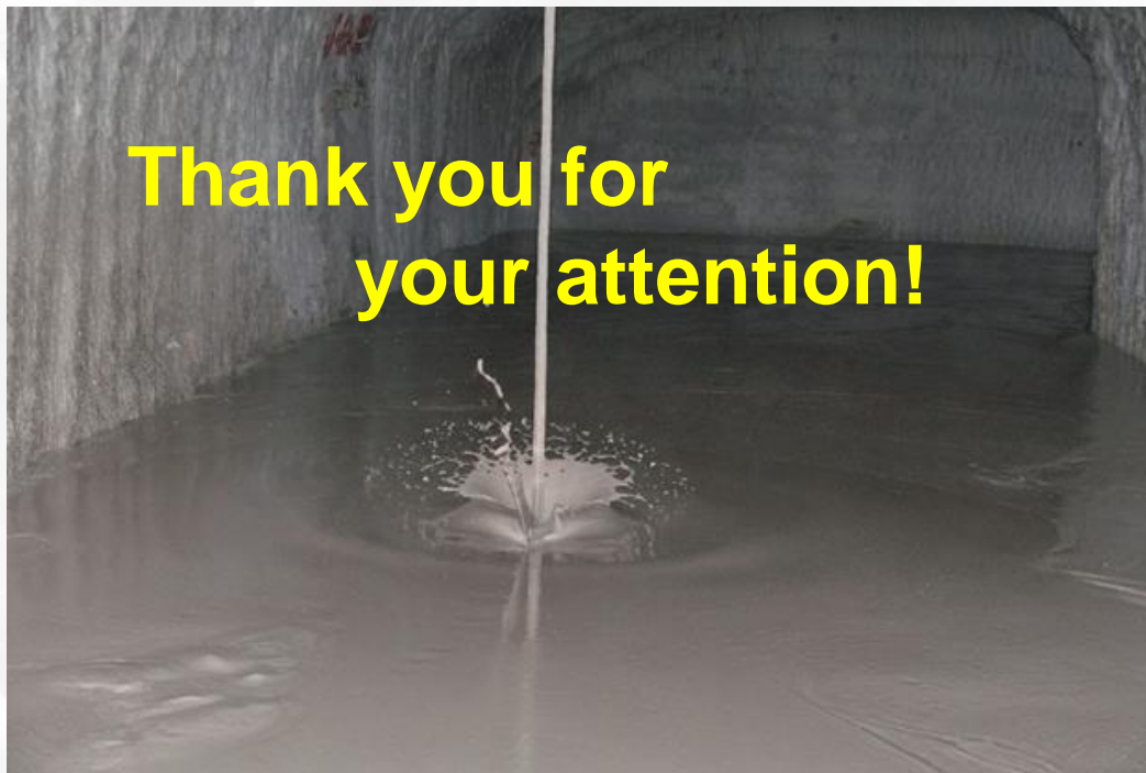
Casting of MgO-Concrete
