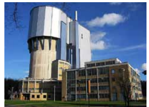
AVR reactor building, status 2007, Jülich (Germany) (source: EWN)
