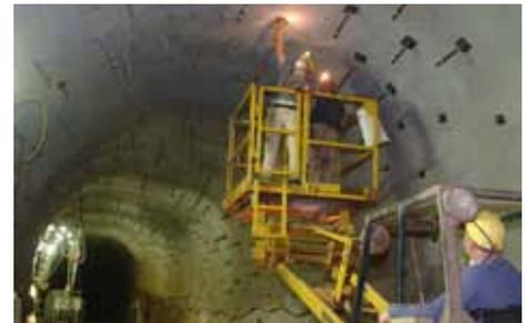
State of the art in constructing drift support systems in clay; the photo shows the roof bolt-shotcrete support system in the Konrad repository (Photo: BfS)
