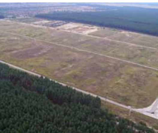
Figure 1: Aerial view of the Buryakovka repository (Ukraine). In front decommissioned parts, in back operating parts of the repository.
