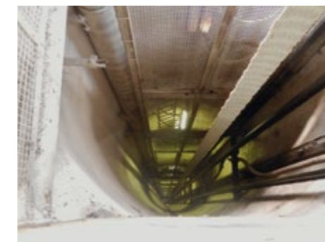
Shaft 1 of the underground laboratory HADES (Belgium)
