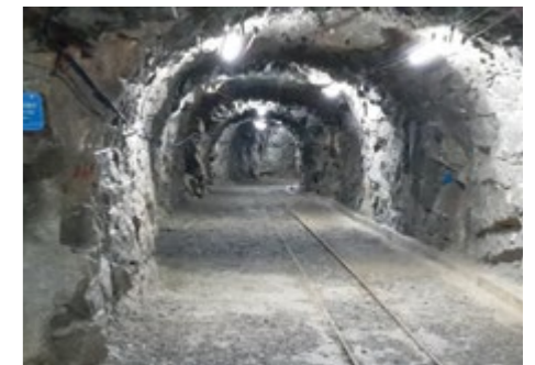
Beishan Exploration Tunnel in granite rock (Gobi Desert, China)
