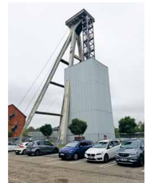
Hoisting tower of shaft Else at Stocamine (France)
