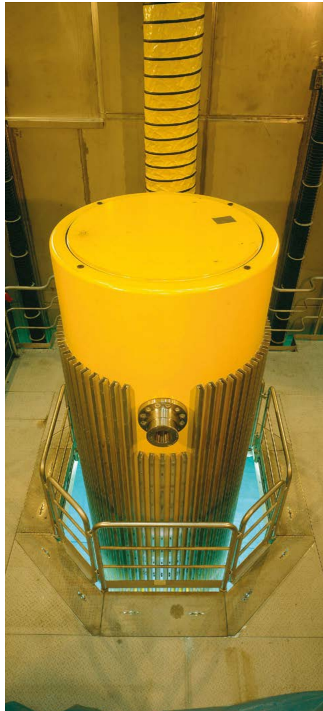
POLLUX® cask for the disposal in rock salt
