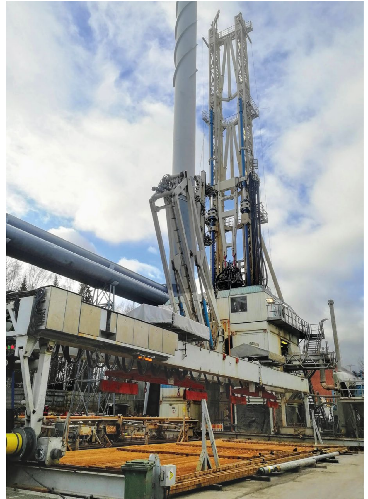
Deep drilling rig in Helsinki (Finland)
