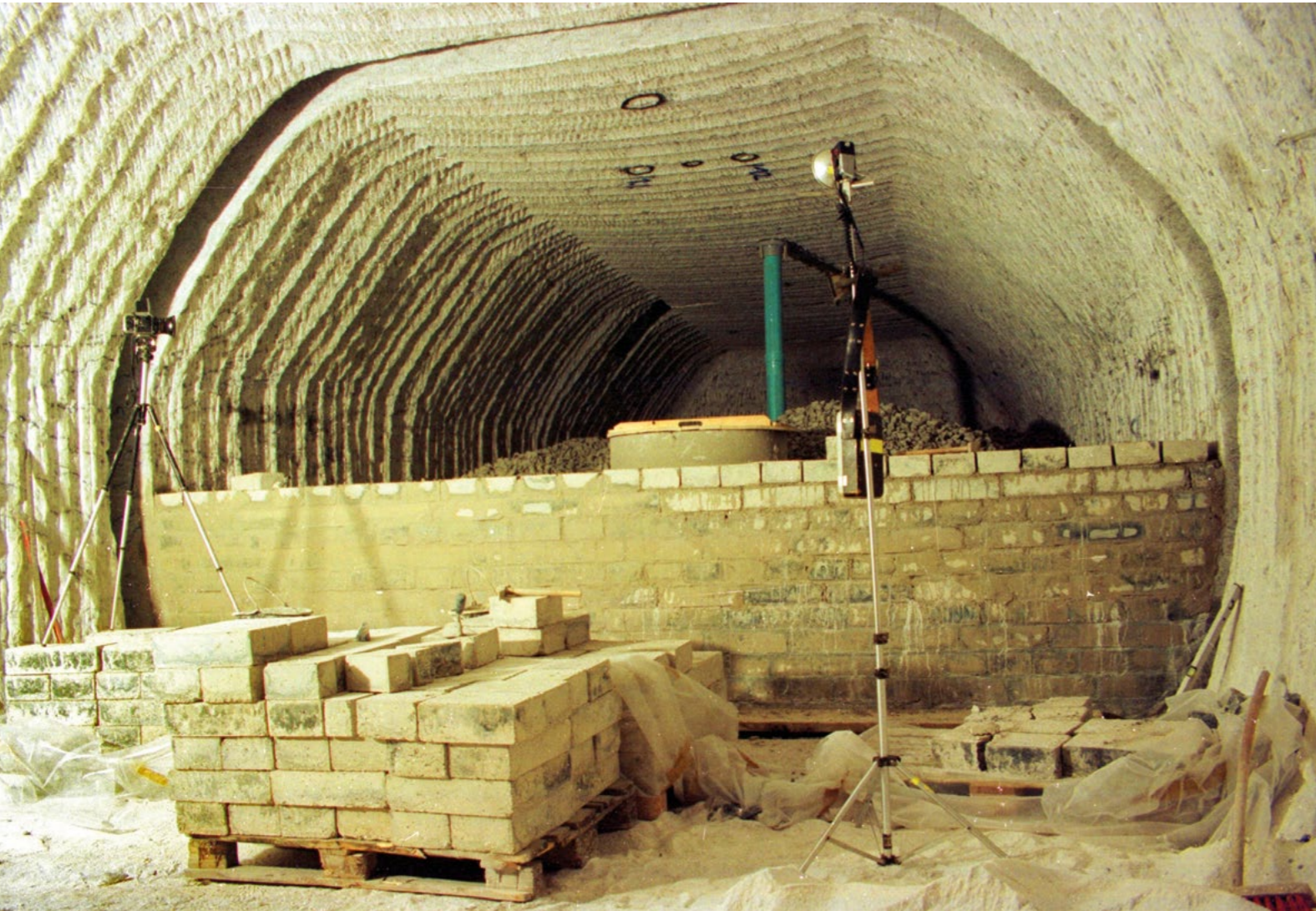
Formwork wall for the construction of a sealing structure, Asse mine
