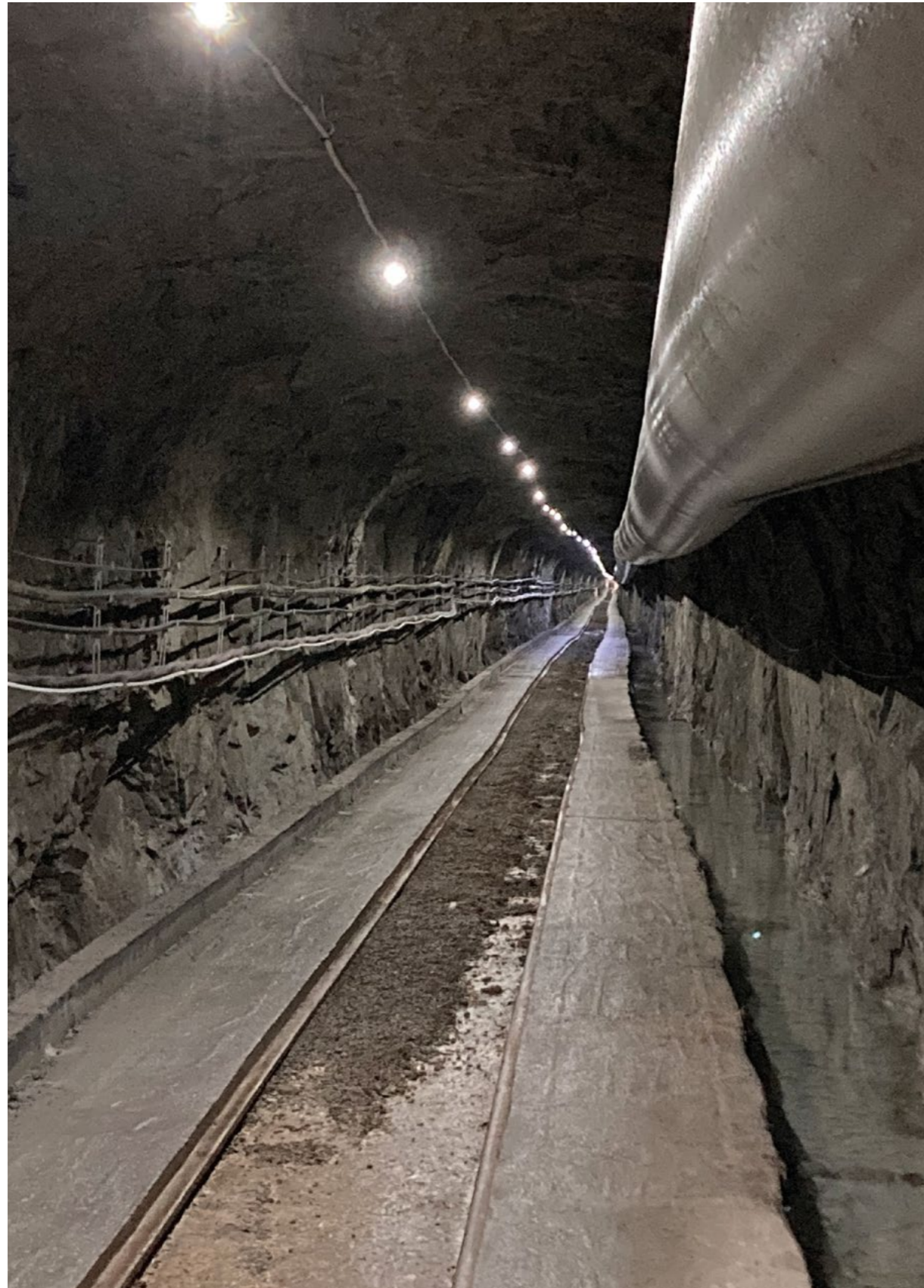
Access tunnel to the Bedretto underground laboratory
