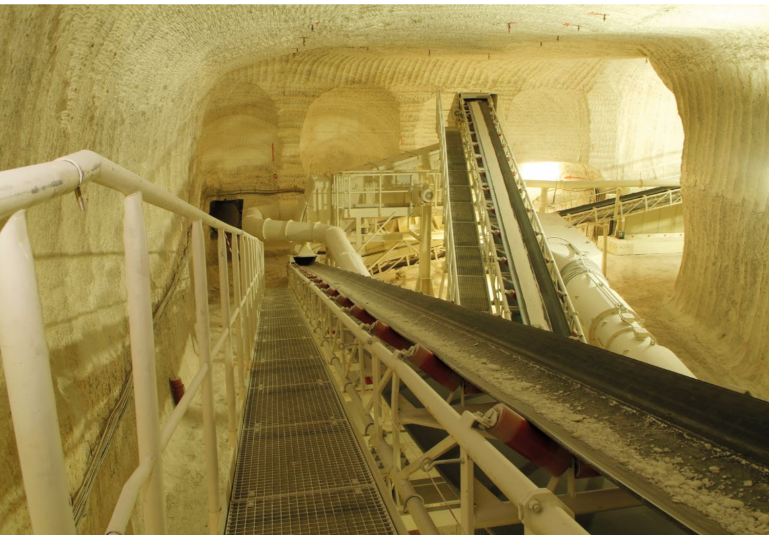
Salt processing plant for the production of soral concrete, Asse mine
