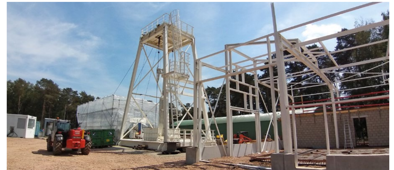
Renovation of the shaft hoisting system of the HADES underground laboratory (Mol, Belgium)
