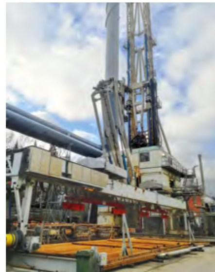
Drilling rig of the world's deepest geothermal borehole in Espoo, Finland
