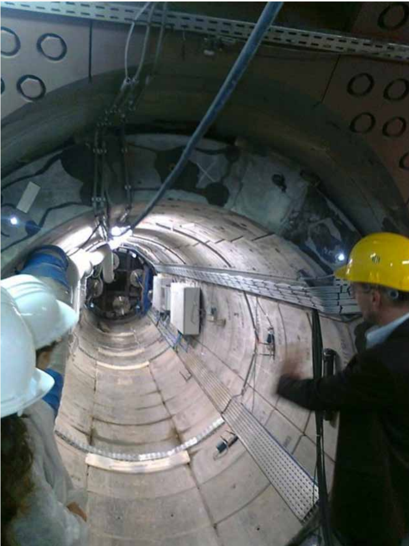
Connecting drift in the underground laboratory in Belgium (Source: ONDRAF/NIRAS)
