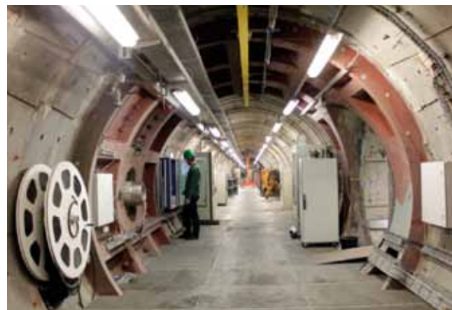
Underground Research Laboratory HADES (Source: ONDRAF-NIRAS)
