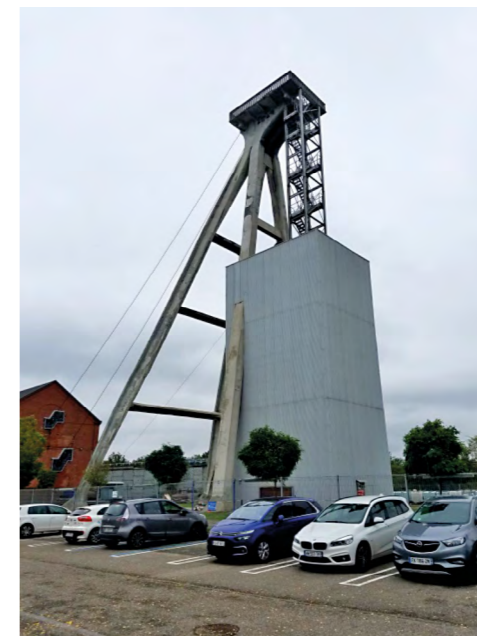
Headframe of shaft Else at Stocamine (France)
