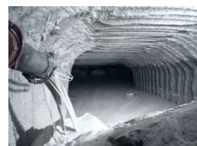
Placing of sorel concrete as mass concrete in the Asse mine
