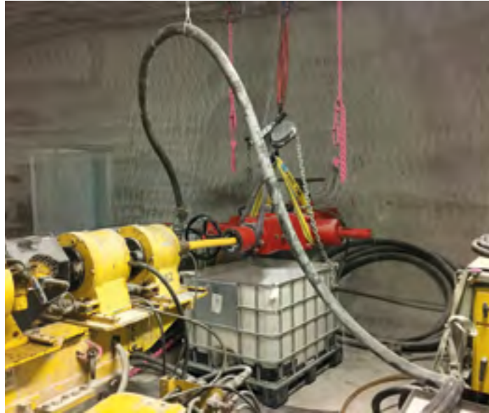
Borehole injections in the Gorleben exploration mine
