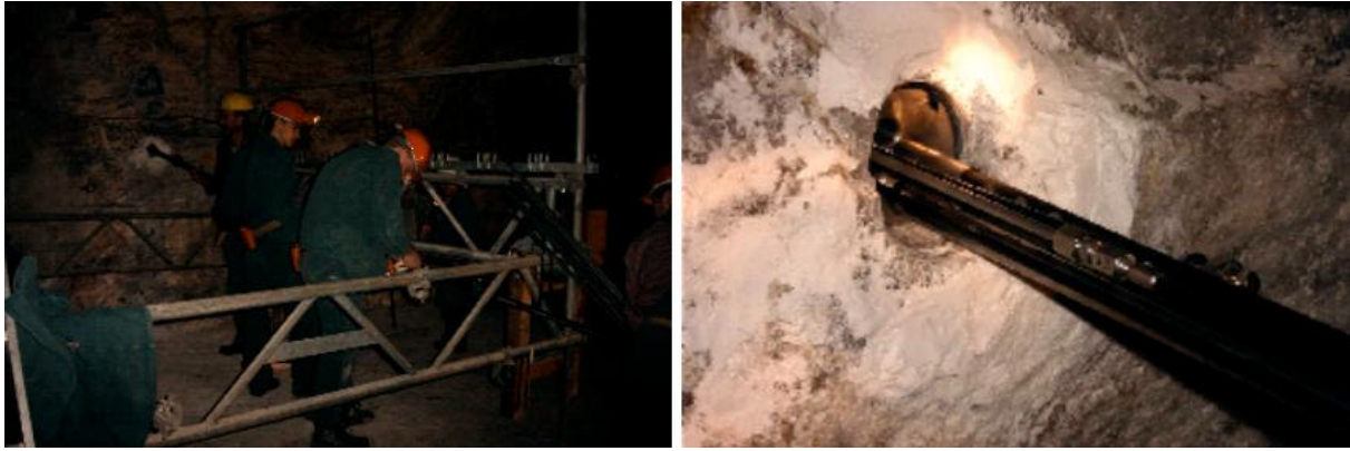
Fig. 3.44: Installation of strain cable
