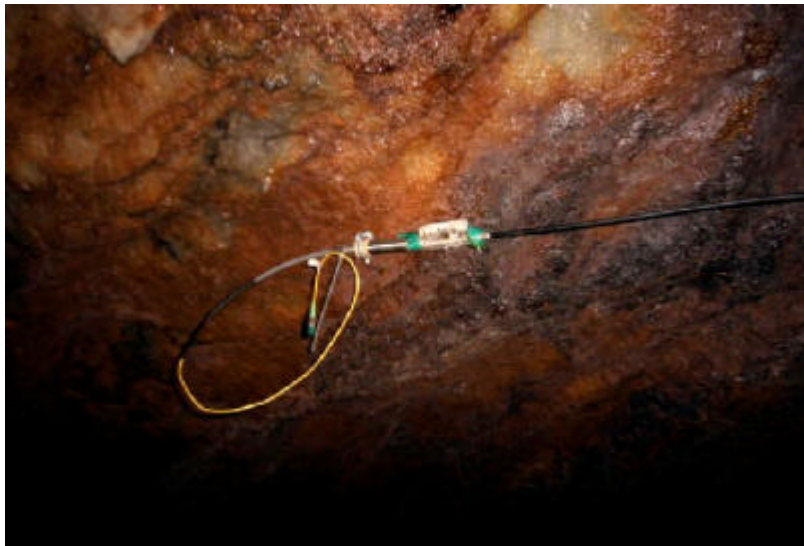
Fig. 3.41: Water leakage sensor SN01102505 equipped with droplet collector
