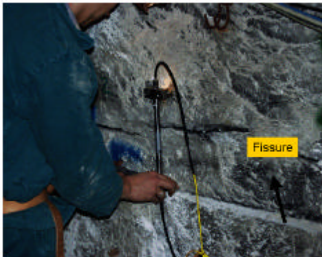
Fig. 4.7: Installation of a fiber optic fissurometer at the Morsleben site
