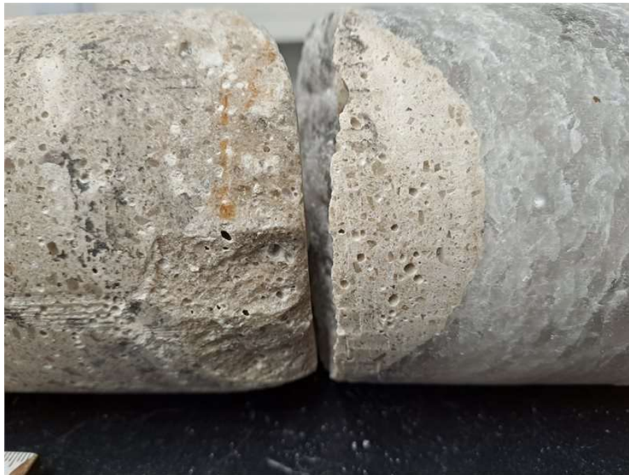
Figure 10 – Core sample of the contact zone between concrete and formation obtained from borehole B23.
