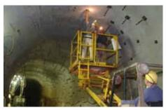
State of the art in constructing drift support systems in clay; the photo shows the roof bolt-shot-crete support system in the Konrad repository (Photo: BfS)
